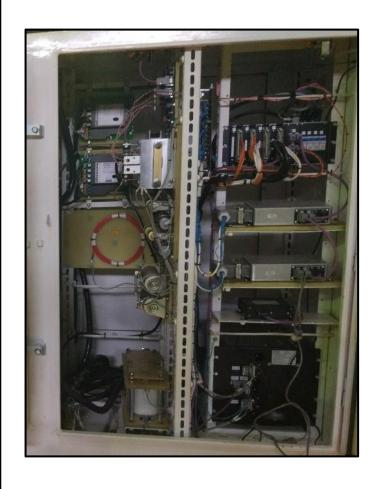
Our new control unit uses thyristor blocks instead of contactors which allows to perform soft electronic switch of the excitation windings of traction electric drives.
