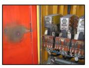
The conventional electric drive control units are based on contactor blocks which are used for excitation windings switching.
